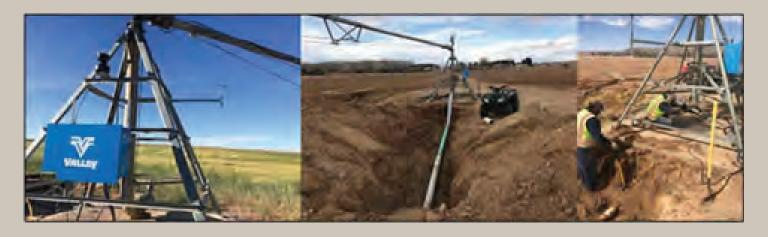
Figure 3. (Left to right). Various stages of electrical grid replacement project completed at ASC Farmington in collaboration with Ross/Wes Electrical Services, Navajo Tribal Utility Authority, and NMSU Facilities and Services. Removing old overhead lines, new buried main lines, new pole and transformers, upgrade from old to new main service panel (far right). NMSU ASC at Farmington 2020.
