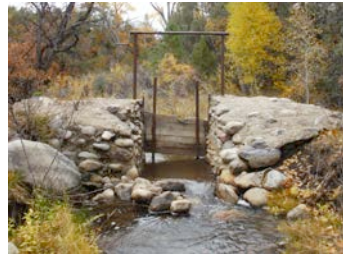
Acequia headgate (photo: Marcos Roybal)
