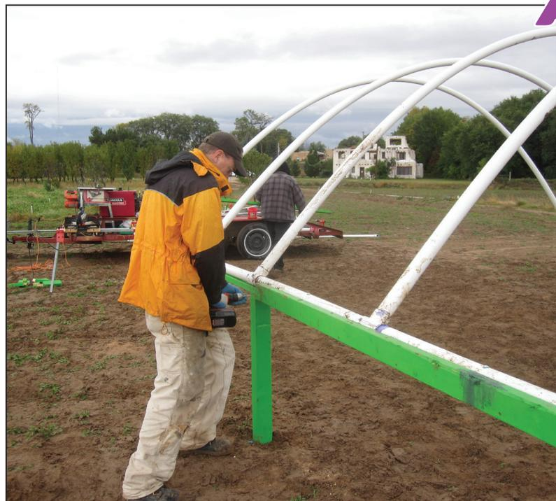
**Figure 19.** Removing the temporary side rail.
