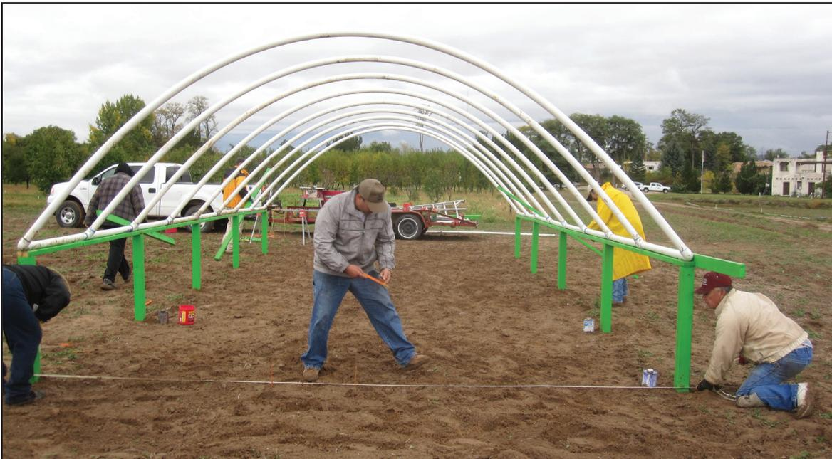
Figure 21. Establishing end wall layout.
