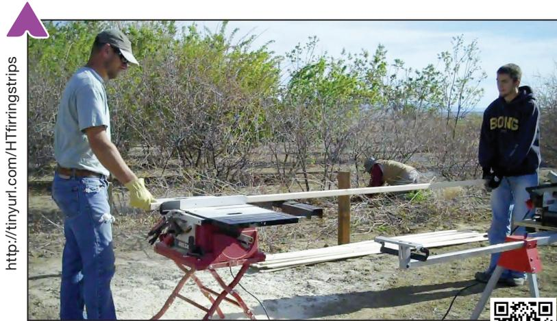
Figure 2. Ripping lath material.
