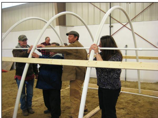
Figure 29. Structural (wooden) and irrigation purlins.
